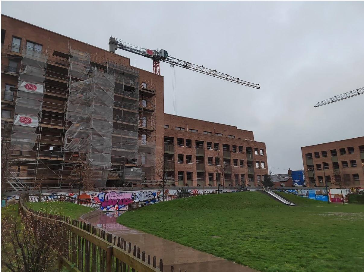
New social housing development in Dublin
