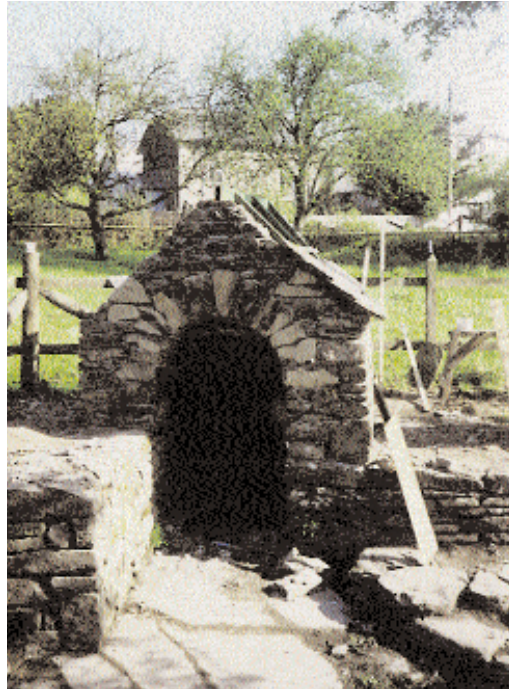
Grant aid project - rebuilt village well (Bryngwyn Women's Institute, Powys-Radnor)
