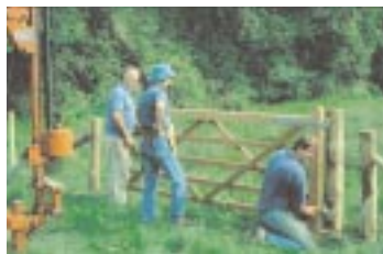
Local contractors working on Tir Cymen farm
